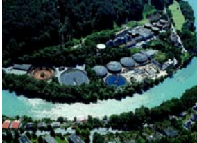
Figure 1: WWTP Bern, Switzerland
