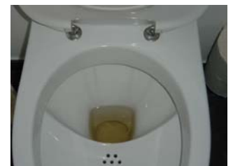
Figure 2: The recycled wastewater shows a yellowish colour
