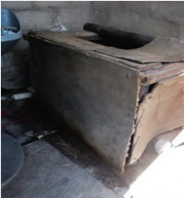
Figure 1: Poor maintenance pedestal.
