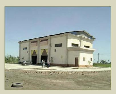
Transfer station at Faraskour, Egypt. The design is suitable for up to 150 tonnes/day capacity
