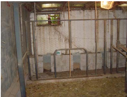
Figure C3: The cinderblock & mortar worm bins are at the back of the chicken house
