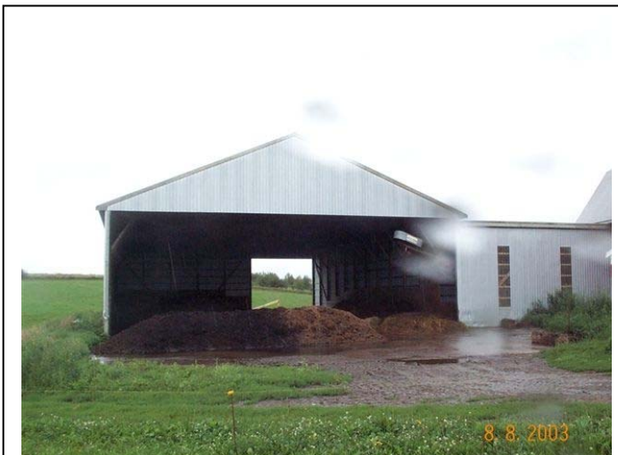
Figure D3: Covered compost pad at Kipawo Holsteins
