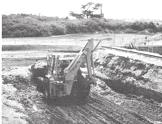
Photo 3: Sludge removal by front-end loader from a batch-operated settling/thickening tank. Achimota FSTP, Accra (Ghana).
