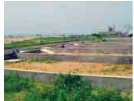
FS plants in Dakar prior to commissioning: (left) settling-thickening tank seen from the outlet end, (right) drying beds for the separated solids.
