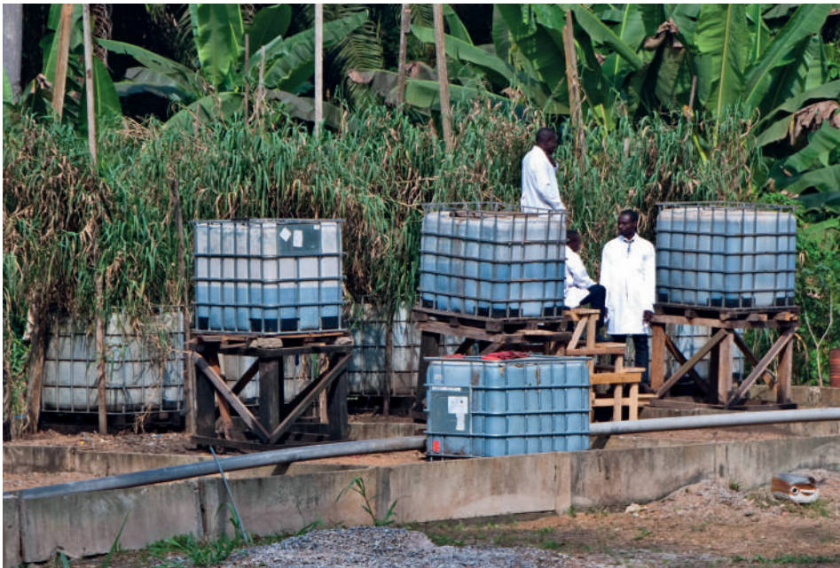
Figure 8.1 Pilot-scale planted drying beds for faecal sludge treatment at the University of Yaoundé I (photo: Linda Strande).
