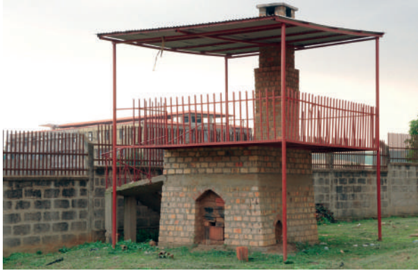
Figure 18.6 FaME (Faecal Management Enterprises) project pilot scale kiln for co-combustion of faecal sludge in brick production in Kampala, Uganda (photo: Pitman Ian Tushemeziwwe).
