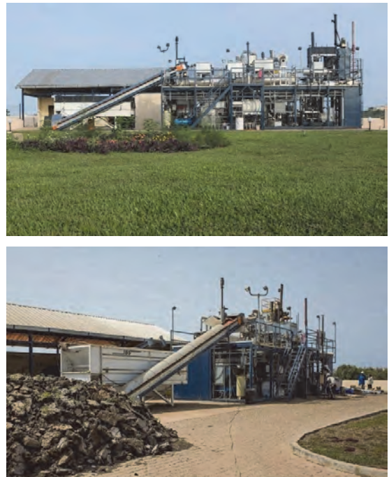
Figure 2.11 The omniprocessor faecal sludge treatment system in operation in Dakar, Senegal (photos: UKZN PRG and Sedron Technologies).
