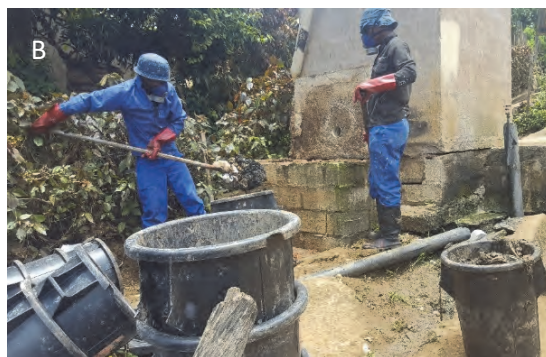
Figure 3.16 A) sampling during a manual emptying operation in Lusaka, Zambia, and B) Durban, South Africa (photos: Eawag).
