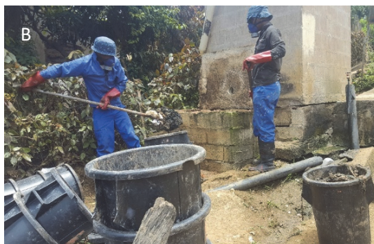
Figure 3.16 A) sampling during a manual emptying operation in Lusaka, Zambia, and B) Durban, South Africa (photos: Eawag).
