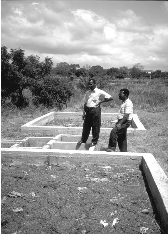
Figure 4 Pilot sludge drying beds in Accra, Ghana
