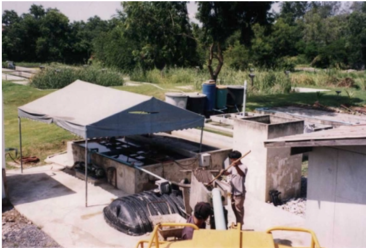
Figure 5. Septage collection in Bangkok and discharging to AIT pilot plant
