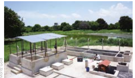
Photo 1: Faecal sludge dewatering research facility at the University of Dar es Salaam in Tanzania.
