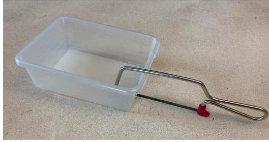
Figure 25: Sawing the cable slot in the short end of the protection box.
