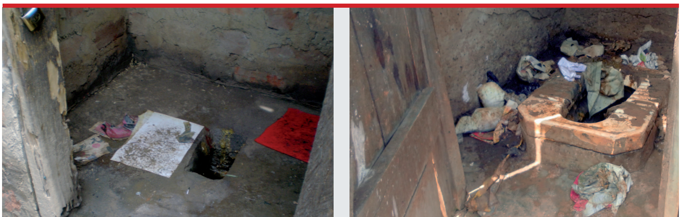
Figure 2: Examples of “unacceptable” hygienic conditions
