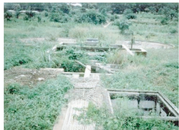
Figures 6.1 and 6.2: Photos highlighting some of the drawbacks of supply-driven sanitation: defunct sewage treatment system, Kumasi, Ghana from the 1970s (top) and an incomplete donor funded latrinisation program, Mauritania, 2004 (bottom). Source: © Sandec
