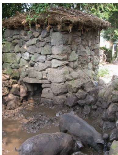
Figure 3.5 Pig-toilet on the island of Jeju, South Korea. The opening in the stone wall is the outlet from the latrine through which the faeces passes for the pigs to consume (Schütze, 2005).
