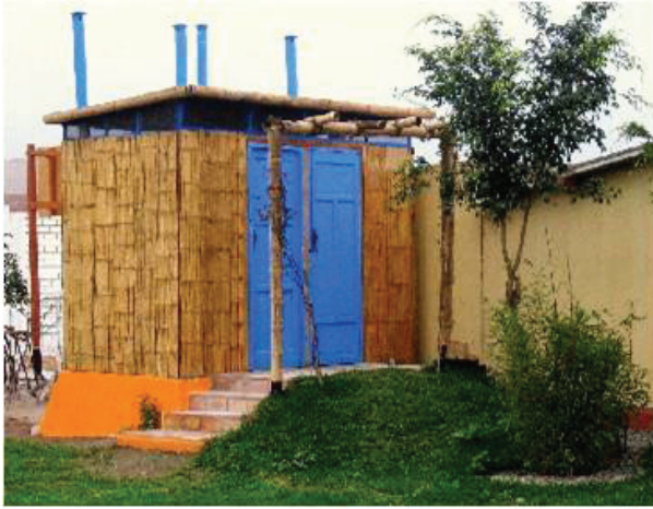
Figure 8.11: Outdoor UDD toilet with gravel filter bed for greywater (bottom right). © Christoph Platzer
