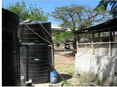
Figure 23: Hanging pipes for the gas transfer.
