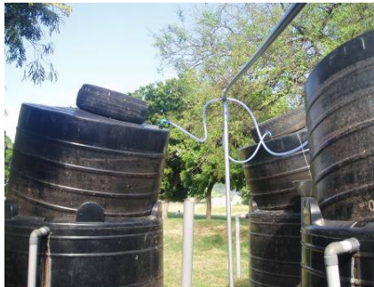
A Original pipes (0.5 inch) were replaced by 0.75 inch pipes. All gas streams were united through a T-cross.
