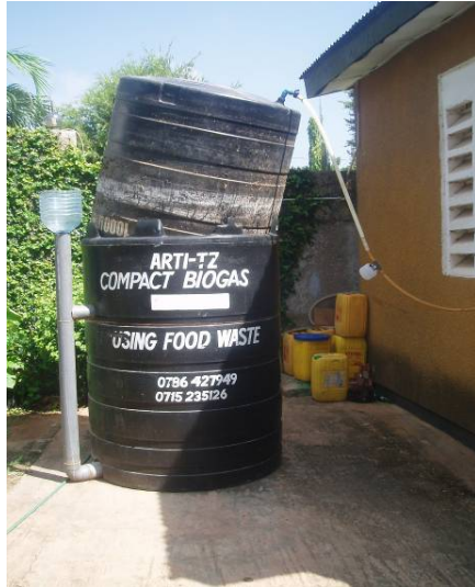
Demonstration plant (household size) at the ARTI office in Dar es Salaam
