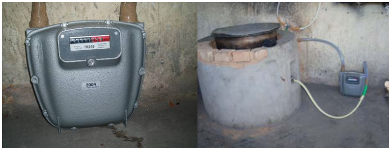
Figure 4: Gas meter provided by Erdgas Zurich (left), gas meter connected to the biogas stove (right)
