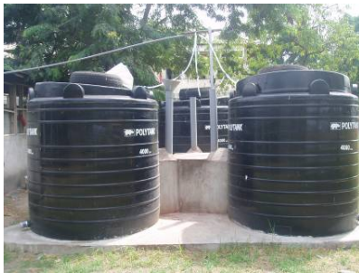
F Gas holders after using biogas, pipes near gas holders straight. VERY IMPORTANT: Even out of the different weight of the tires by help of sand bags.
