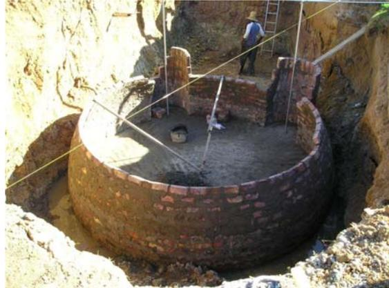
**Picture 6:** When the wall reaches a certain height respectively a certain slope hooks are required to hold the bricks in position (25.11.2008).
