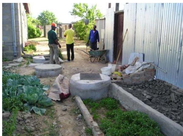
**Picture 15:** Dome inlet, gas outlet, and dome outlet chamber and an expansion chamber (in front). Expansion chambers have been installed in older systems, for agricultural purposes.
