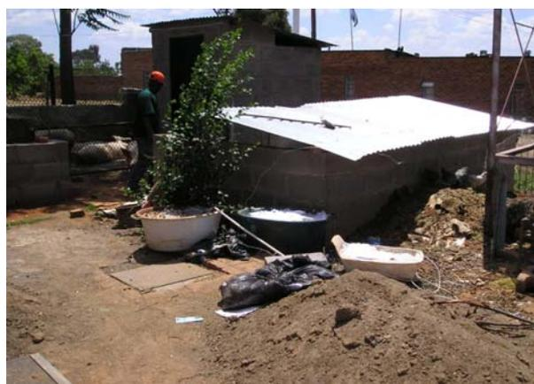
**Picture 11:** Dome inlet and outlet (lower left corner) in the front. In the background the open stable for the pigs. Pig waste water is directly flowing into dome inlet chamber. Two bowls of feedstock paper are standing next to the inlet chamber.
