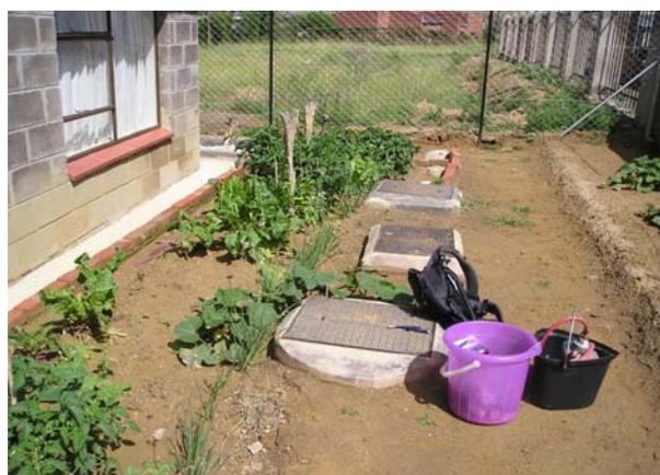
**Picture 3:** Dome inlet, gas outlet, and dome outlet chamber in front of the ABR (all in a line).
