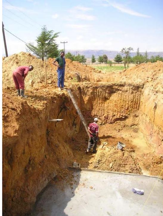
**Picture 2:** The foundation for the digester is already casted while the one for the ABR is still in preparation. Final digging and soil removal has to be done manually (21.11.2008).
