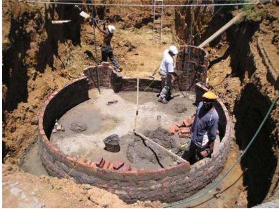
**Picture 5:** The positions of inlet and outlet chamber depend on the existing sewage pipe and the available space for ABR and PGF (25.11.2008).
