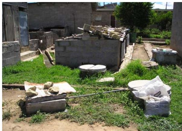
**Picture 9:** Gas outlet, dome inlet and outlet in the front. In the background the open stable for the pigs. Pig waste water is directly flowing into dome inlet chamber.
