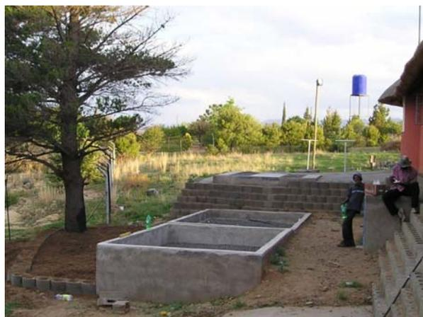
**Picture 6:** View from opposite side. Two PGF-beds in front of the terrace (including ABR and digester).
