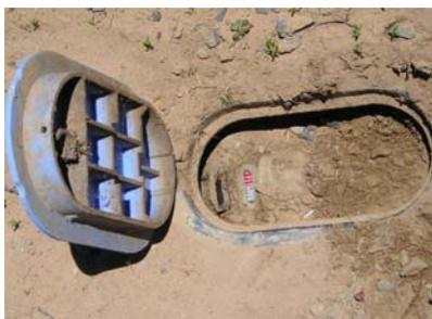
**Picture 22:** Water meter. Freshwater consumed by the household is measured.
