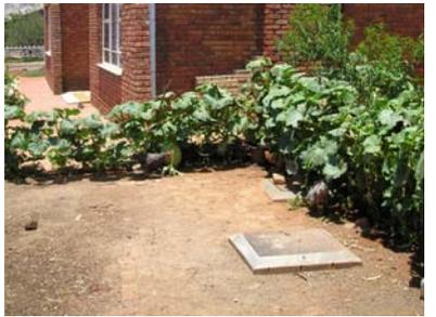
**Picture 7:** Gas outlet and dome outlet chamber covered with plants (13.1.2009).
