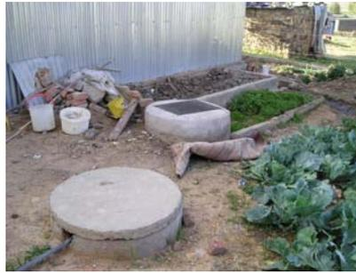
**Picture 2:** Gas outlet and dome outlet in the back (Nov. 2008)
