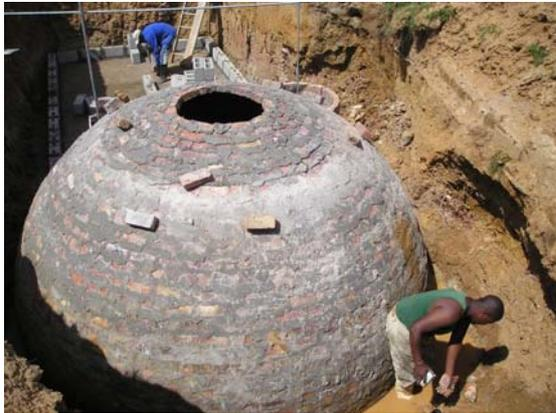
**Picture 7:** Hooks weighted with additional brick (hanging on the wall) keep the placed bricks in position (2.12.2008).
