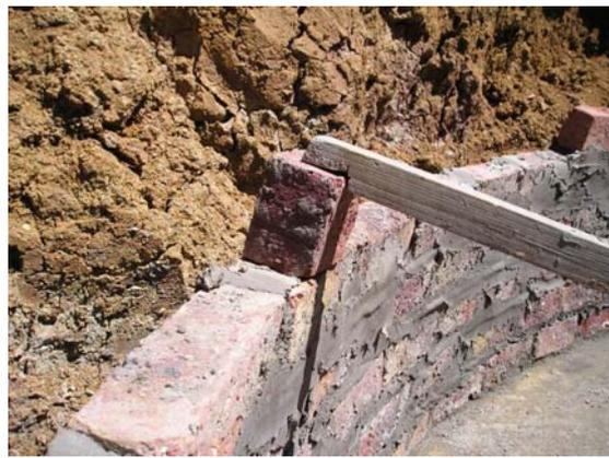
**Picture 4:** The wooden lath got a rectangular cut in order to easily keep the bricks in the right position (25.11.2008).
