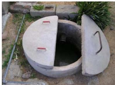
**Picture 5:** Dome inlet, black waster mixed with chicken waste (Nov. 2008).
