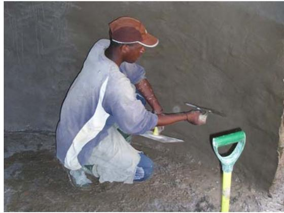
**Picture 12:** The digester is smoothly plastered from inside from the top to the bottom. Afterward the curing process starts (12.12.2008)
