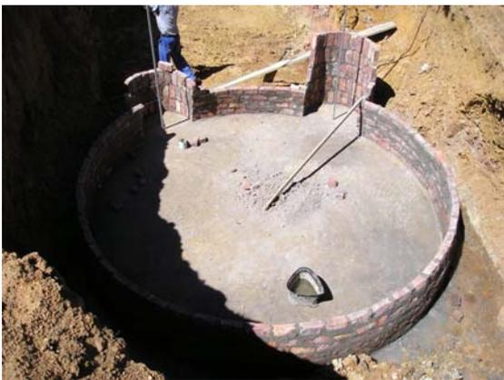
**Picture 3:** The first rows of the digester are built. The circular form is made with a lath that is attached in the middle of the foundation (radius, 25.11.2008).
