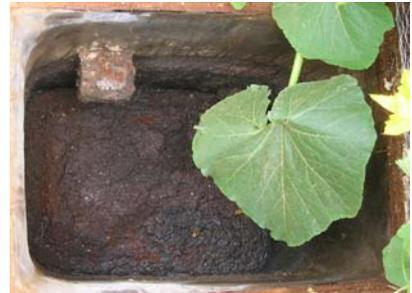
**Picture 9:** Dome outlet with scum layer (Nov. 2008).
