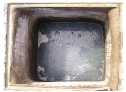
**Picture 12:** Dome outlet, organic solids remain within the digester and get decomposed (8.1.2009).
