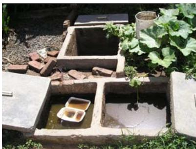
**Picture 10:** Outlet chambers of PGF, effluent used for irrigation (13.1.2009).
