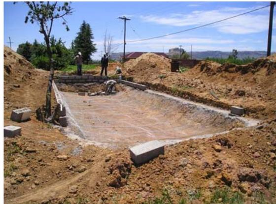
**Picture 14:** The PGF is build up in order to provide a post-treatment of the effluent (7.1.2009).
