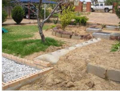
**Picture 2:** Chambers of digester, ABR and PGF (left) (Nov. 2008).
