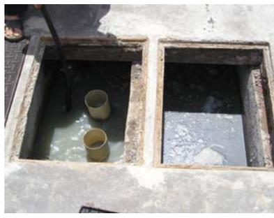
**Picture 8:** Two chambers of ABR. Two pipes that lead to water to the bottom of the chamber (Nov. 2008).
