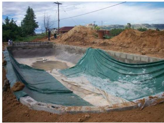
**Picture 16:** In order to protect the plaster from sunlight it gets covered. Too much sunlight causes a fast drying of the plaster resulting in generating breaks (leakages, 13.1.2009).
