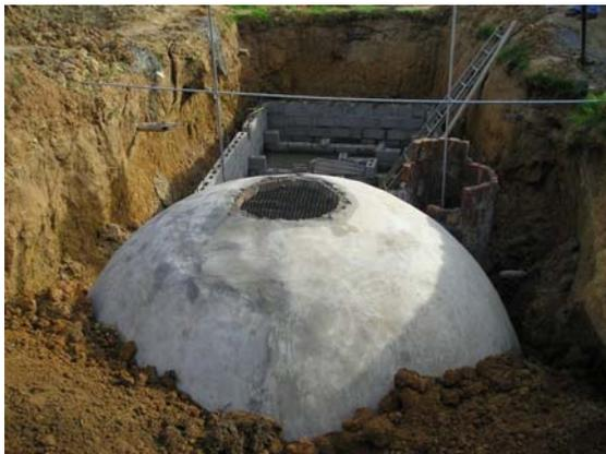
**Picture 9:** Before closing the upper part of the digester it gets smoothly plastered and partly covered with soil (8.12.2008).
