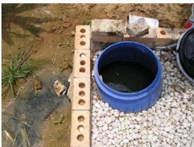
**Picture 10:** Effluent tank in PGF, used for irrigation (1.9.2009).
