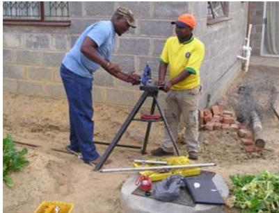
**Picture 4:** Gas meter gets installed. Pipes are cut (19.11.2008).
