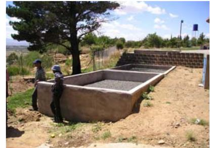
**Picture 3:** PGF in series; different size of crashed stones (Nov. 2008).
