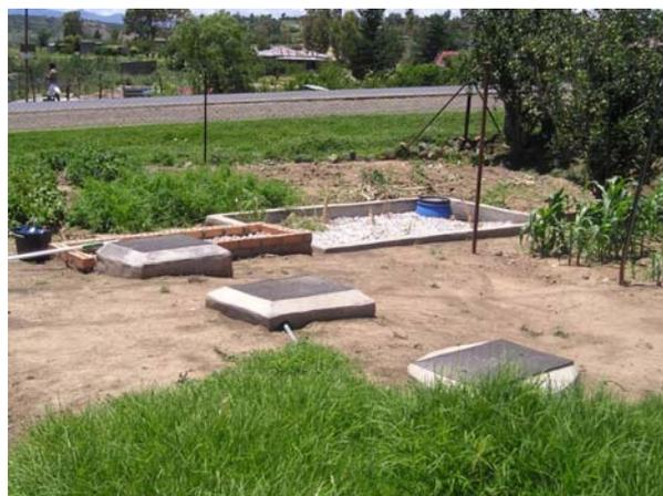
**Picture 13:** Dome inlet, gas outlet, and dome outlet chamber in front of the ABR and PGF.
