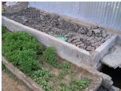
**Picture 4:** Drying bed, effluent is put on top to be dried (Nov. 2008)
