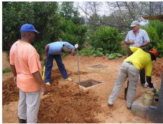
**Picture 4:** Here the gas pressure was build up manually by blowing air into the digester. This could also be done with exhaust gas of the car. Filling the inlet with water also increases the gas pressure to a certain extent (the higher the pressure the easier the detection is).
