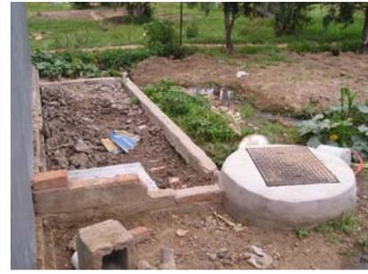
**Picture 3:** Drying bed on top of expansion chamber (10.12.2008).
