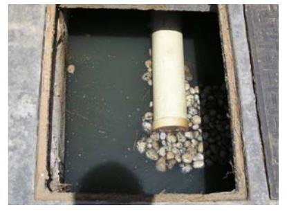
**Picture 9:** Last chamber of ABR; effluent is entering the connection pipe to PGF (Nov. 2008).
