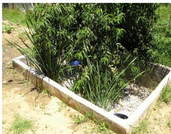
**Picture 2:** The PGF including the effluent collection tank in the lower corner (partly visible).
