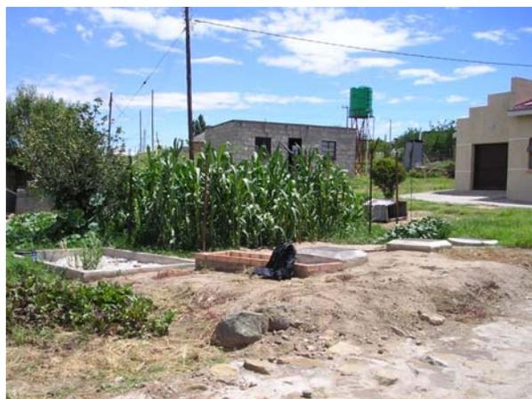
**Picture 14:** Biogas system in front of maize field that gets irrigated with effluent. On the right hand site part of the owners building where biogas is used.
