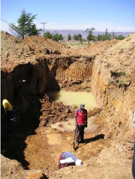
**Picture 1:** After locating the site the soil is dug out according to the project plans. In the foreground the hole for the digester and the ABR is visible, in the background for the PGF (17.11.2008).
