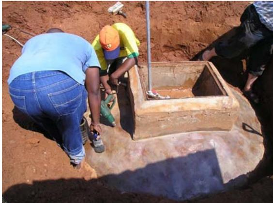
**Picture 7:** After detecting the leakages the leakage points have to be marked. Then the surface gets dried and then sealed with hot (melted) candle wax that enters the capillary tubes.
