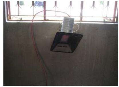
**Picture 6:** Gas heater operated with biogas (Nov. 2008).
