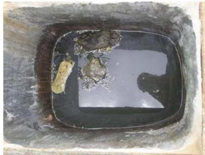
**Picture 8:** Dome outlet, some sanitary towels passed the digester (9.1.2009).
