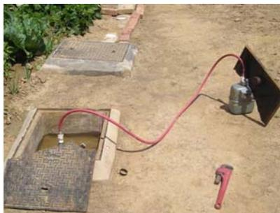
**Picture 7:** During gas flaming the iron plate protects the pipe (18.12.2008).
