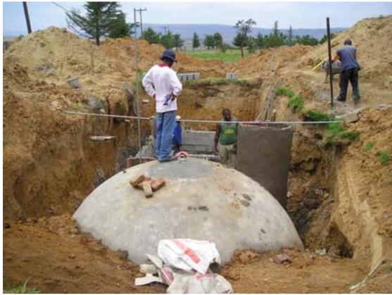
**Picture 11:** The digester is closed by installing a gas plug valve where the gas can be released. The inlet chamber is going to be finalized (10.12.2008).
