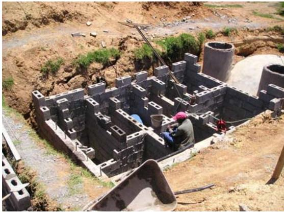
**Picture 13:** Inlet and outlet chamber, as well as ABR are going to be finalized (7.1.2009).
