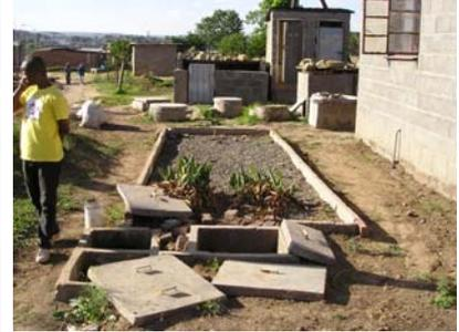
**Picture 3:** PGF with outlet chambers (Nov. 2008).
