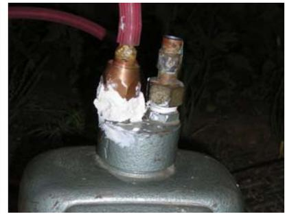
**Picture 6:** The pipe is gas tightly connected. Sealing wax is attached (8.12.2008).
