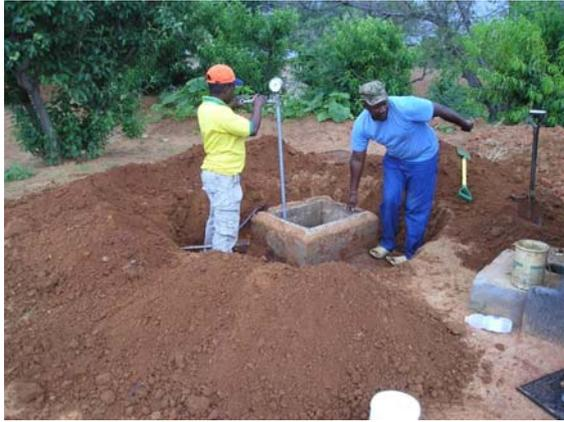
**Picture 5:** The next step consists of testing the surface of the gas storage chamber. Therefore part of the digester has to be dug free.
