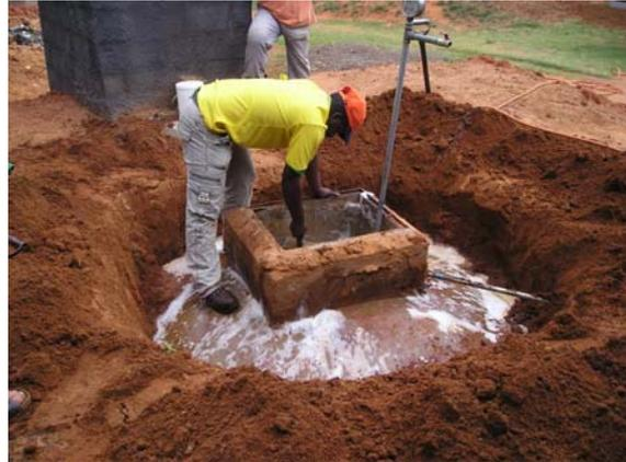
**Picture 6:** Testing is also done with soap water. Again air has to be blown regularly into the digester in order facilitate the detection.
