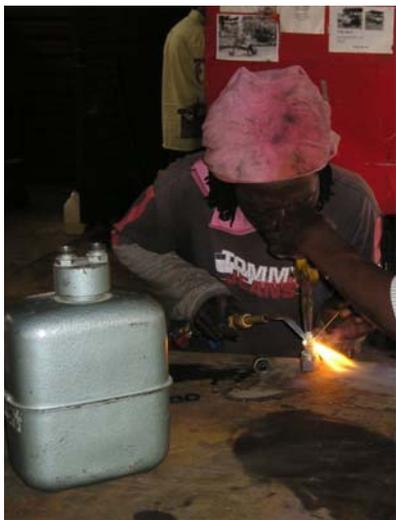
**Picture 19:** Connections for gas meter are soldered. Prefabricated connection pieces that fit to gas meter were missing.
