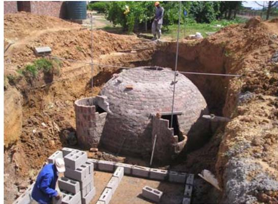
**Picture 8:** Besides finalizing the digester the ABR is built up (foundation and first brick rows can be seen in the front, 2.12.2008).
