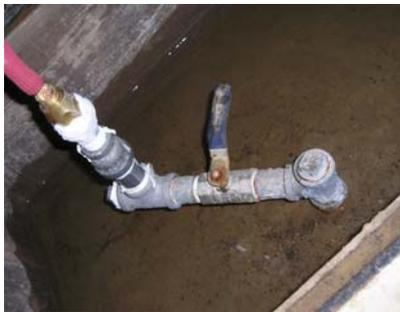
**Picture 4:** Gas plug valve (closed) is connected with plastic pipe (8.12.2008).
