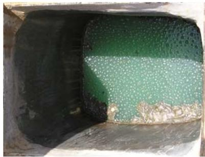
**Picture 5:** Dome outlet, no biogas production (Nov.2008)
