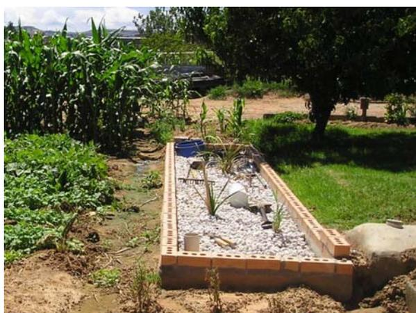
**Picture 8:** Part of ABR (on the right) and PGF. At the upper end of PGF the collection tank (blue) is stored in the corner.
