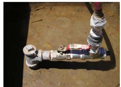
**Picture 12:** Open gas valve with connection to gas meter (9.1.2009)
