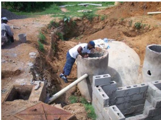
**Picture 15:** Inlet chamber gets connected with waste water pipe from school (12.1.2009).
