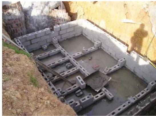
**Picture 10:** The chambers of the ABR are visible. The walls are reinforced with steel rods that are put into the brick holes and then filled with plaster (8.12.2008).
