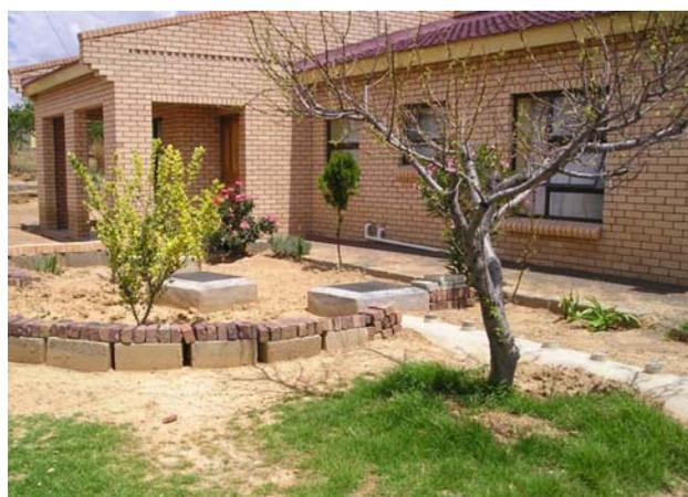
**Picture 7:** Gas outlet, dome outlet and ABR.
