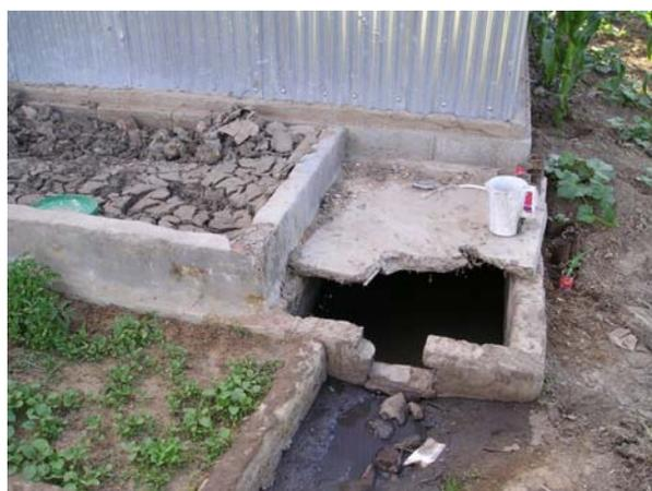
**Picture 16:** Expansion chamber outlet, it overflows automatically as soon as a certain water level is reached, then enters the distribution canal and irrigates the garden.
