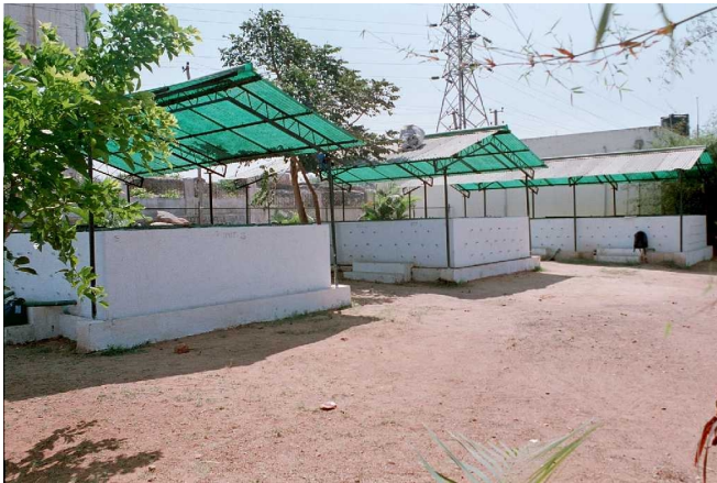
Figure : Composting bins at Kalyana Nagar, Bangalore
