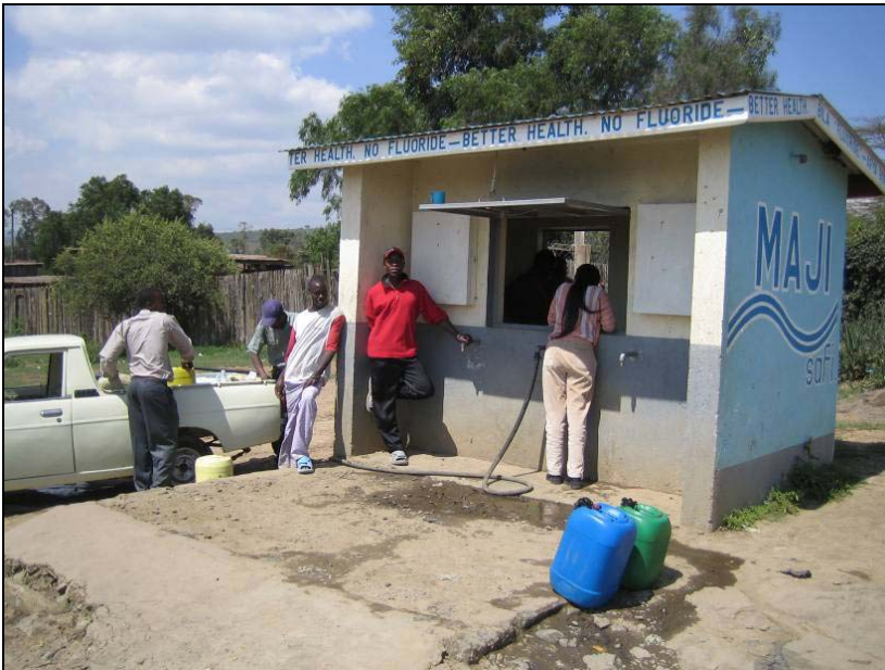
Figure 6-2: Water kiosk in Naivasha that sells defluoridated water from a community filter installed by CDN WQ. The water kiosks are opened at fixed times that are set by the local water management.
