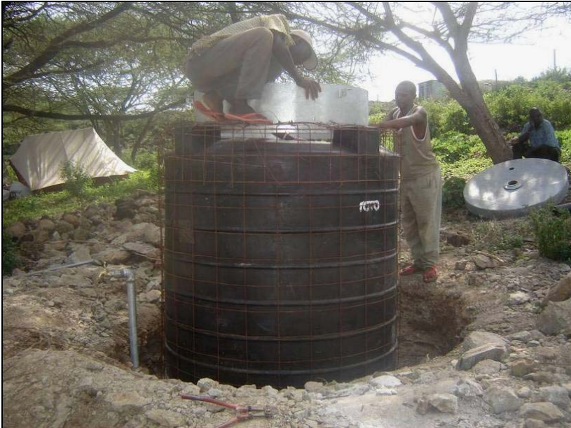
Figure 6-1: Remote community filter under construction. The concrete walling will protect the PVC tank from damage.
