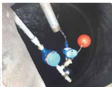
Photo 2: Aquatabs Flo chlorinator.
