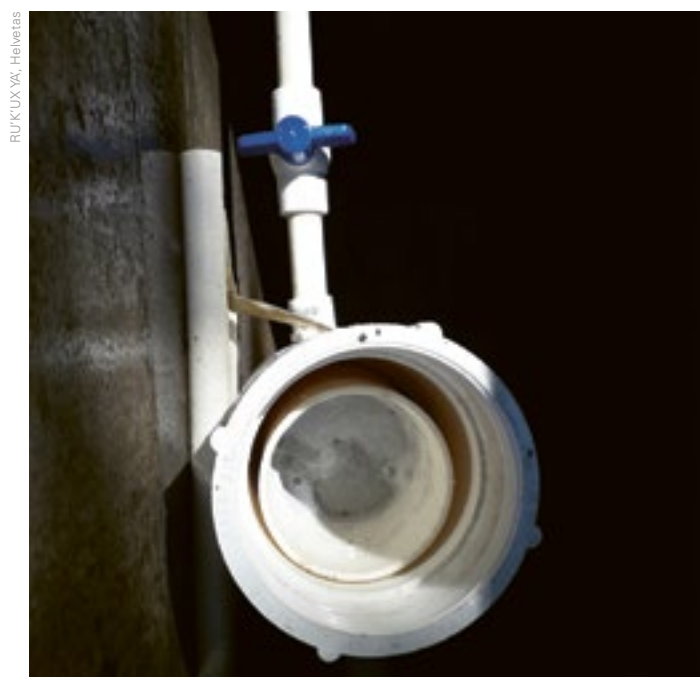
Photo 1: View of the A'Jín chlorinator in use.
