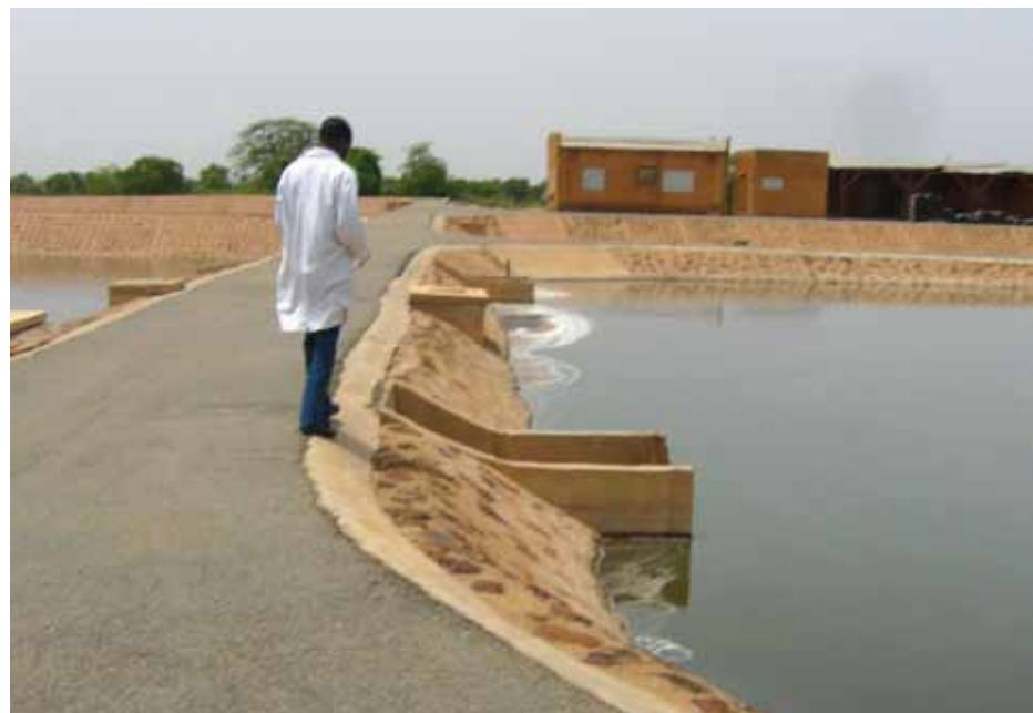
Photo 1: ONEA's chemist taking samples in the second anaerobic basin at the WSP in Ouagadougou, Burkina Faso.
