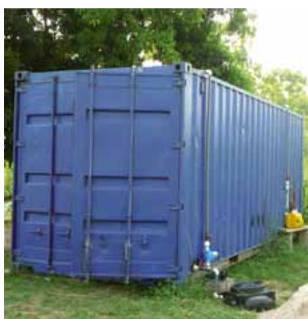
Photo 1: Used shipping container currently converted into a biogas digester at KNUST, Kumasi, Ghana.
