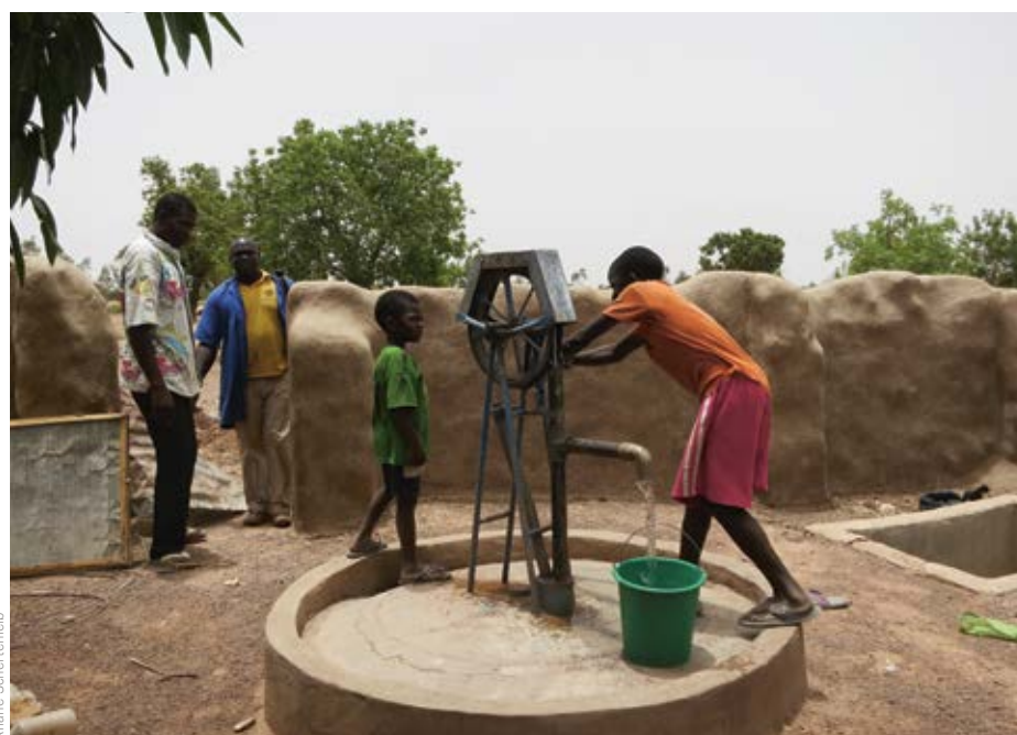
Photo 1: Upgraded well with rope pump on premises.
