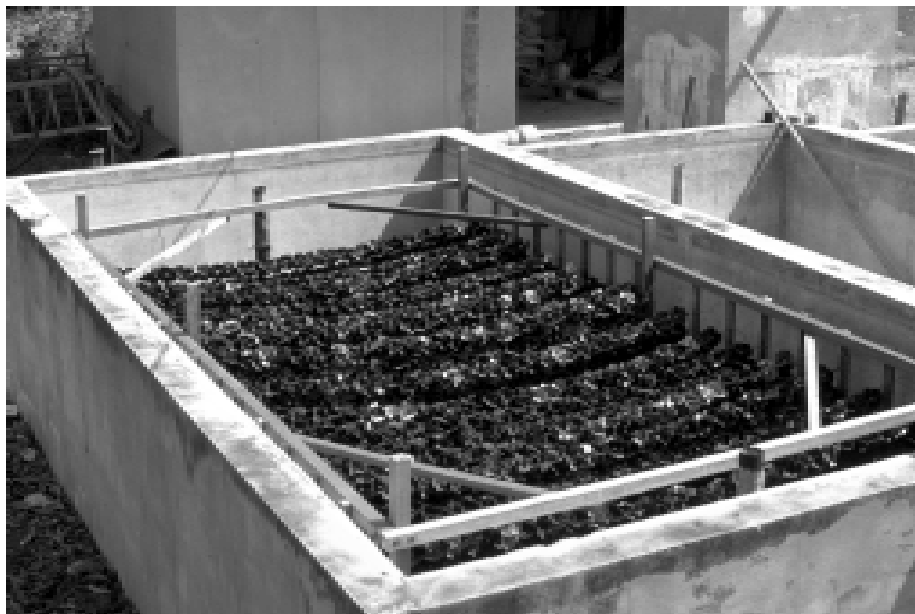
Plastic modules in the attached-growth waste stabilisation ponds at AIT, Bangkok. The ponds are used to polish the percolate from the planted septage drying beds (Photo: Thammarat Koottatep)
