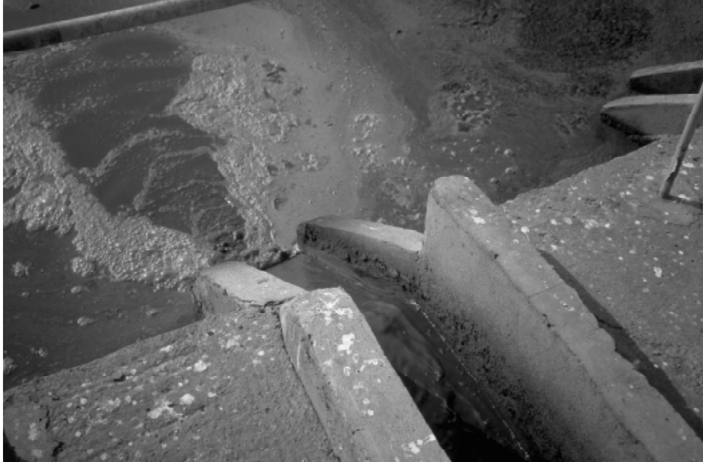
Fig. 2 Supernatant from a FS settling tank overflowing into an anaerobic pond at the Achimota FSTP in Accra, Ghana. What standards should be established and how many ponds in series are required to meet these standards?
