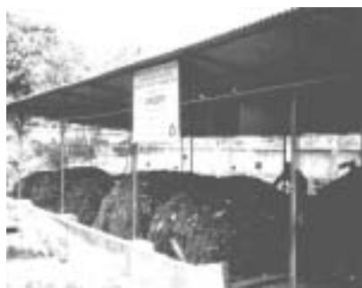
Fig. 2: Mirpur composting shed, Dhaka, Bangladesh (photo Isabelle Rytz)
