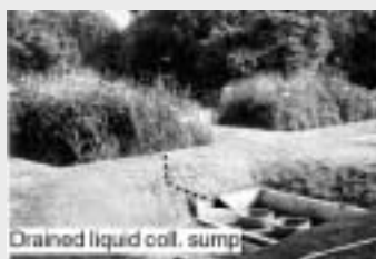
Drained liquid coil sump
