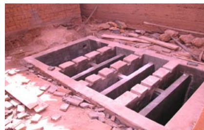
Figure 4: Two ABRs were installed in Shaxi Town according to the outcomes of the research conducted in Hanoi and Bangkok
