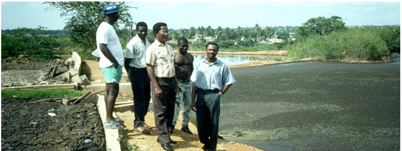
Photo 5: Ghanaian sanitation experts and treatment plant operator at an FS treatment plant in Ghana (left: FS settling-thickening tank; right: stabilization pond for settling tank supernatant)
