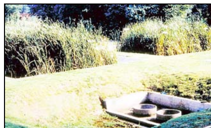
Photo 1: Cattail-planted constructed wetlands
