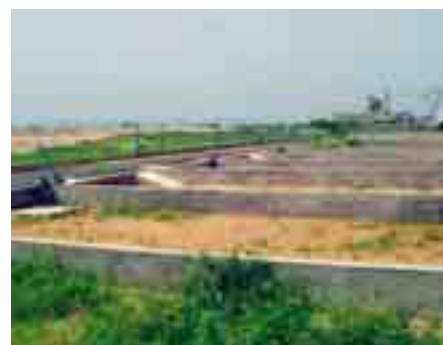
FS plants in Dakar prior to commissioning: (left) settling-thickening tank seen from the outlet end, (right) drying beds for the separated solids.
