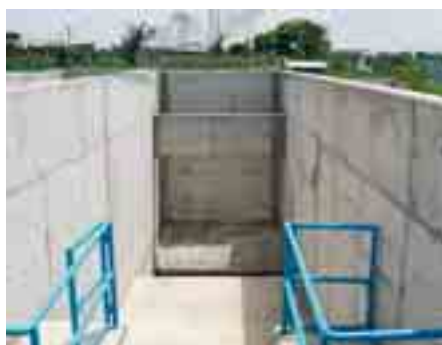
FS plants in Dakar prior to commissioning: (left) settling-thickening tank seen from the outlet end, (right) drying beds for the separated solids.
