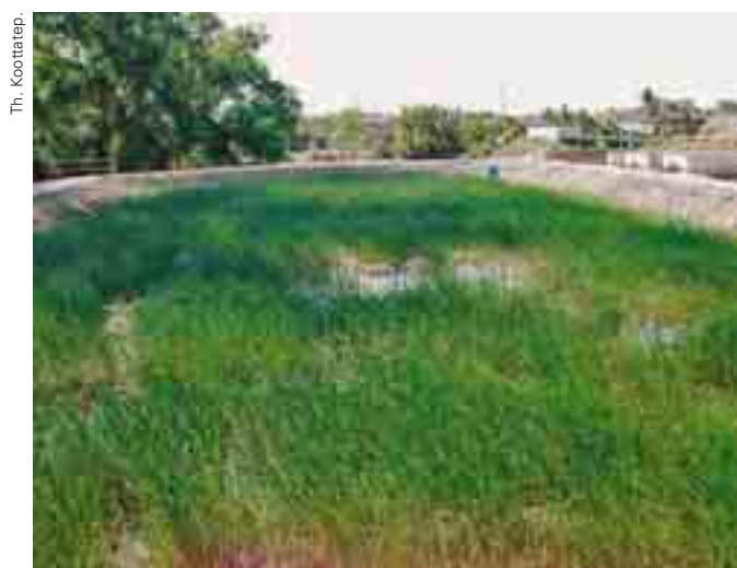
Photo 2: Wastewater treatment plant comprising an anaerobic baffled reactor, a constructed wetland and three sludge drying beds in Songkla Province, Thailand. The system treats domestic wastewater of 50 households.
