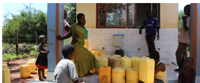
(b) Final installation (outside the water kiosk)
