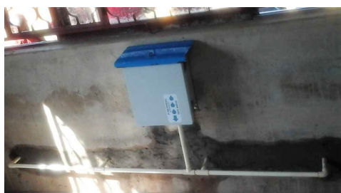
(a) Initial installation (inside the water kiosk)
