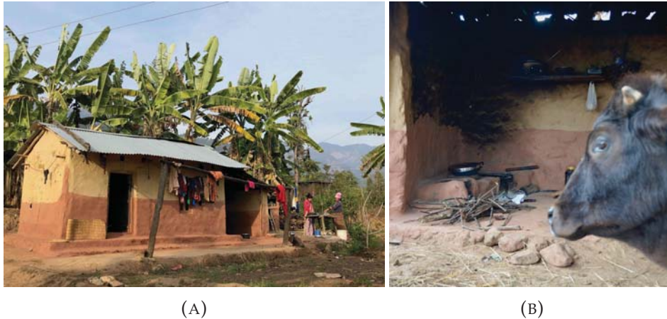
FIGURE 3.1: Household with a fireplace to cook outside, a washing station, walls build from stones and mud, CGI sheets on the roof (A) and kitchen in proximity to animals (B).
