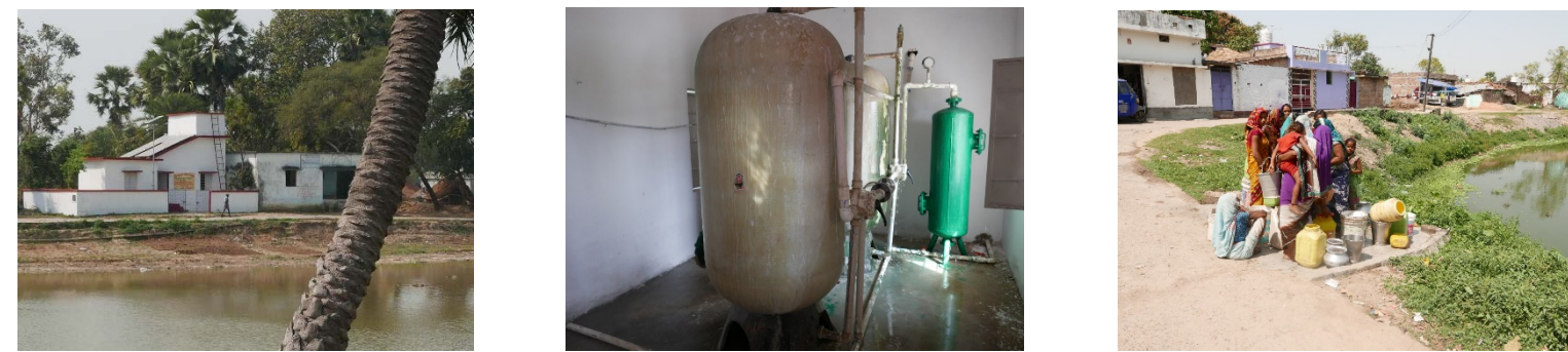
Fig. 1b. Community-based water scheme. Left: Pump & Filtration house. Middle: Arsenic filtration unit in the Filtration house. Right: Public collection tap of the piped water distribution scheme.
