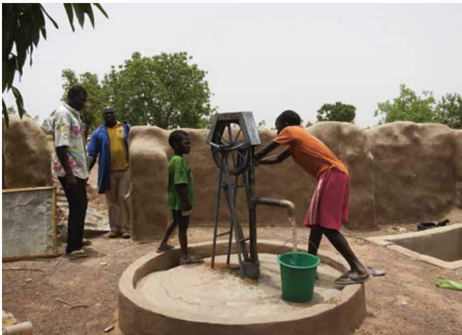
Photo 1: Upgraded well with rope pump on premises.
