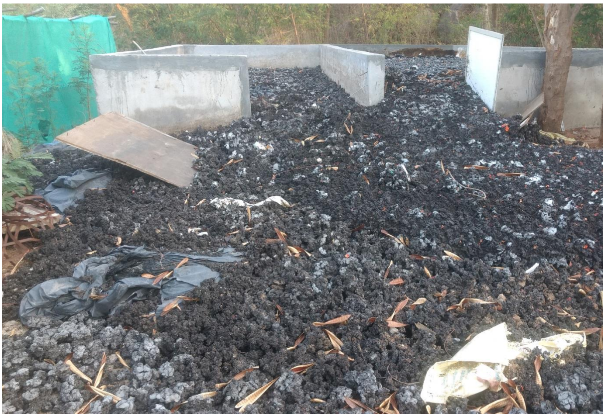
Figure 5: Solids management issues at an SSS system (Photo: Shreyas Kumar).
