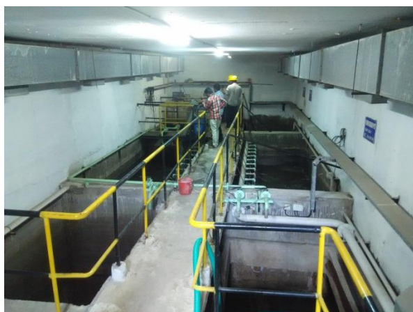
Figure 15: Due to space constraints and the infeasibility of structural modifications, retrospective upgrades may not be realistically possible for SSTPs (Photo: Shreyas Kumar).
