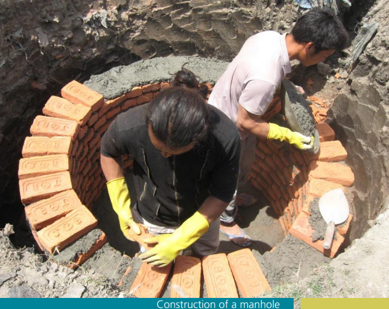
Construction of a manhole
