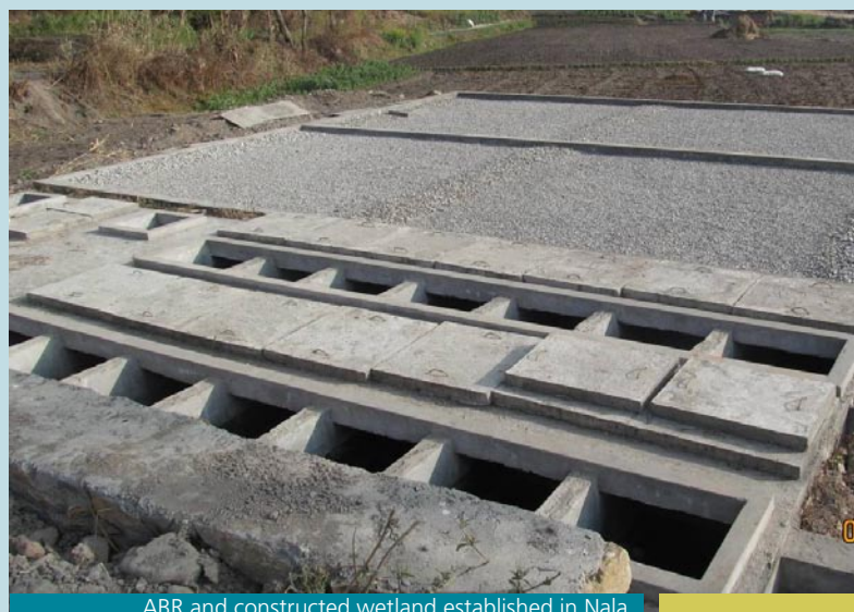
ABR and constructed wetland established in Nala
