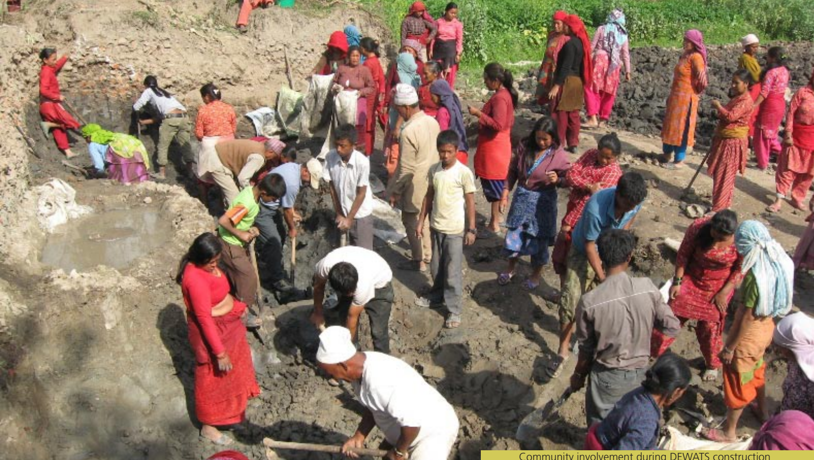
Community involvement during DEWATS construction
