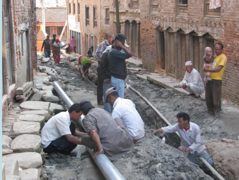
Construction of simplified sewer lines
