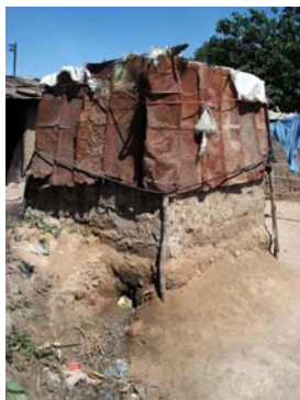
Image 1: Simple pit latrine in Chang'ombe
