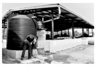
Photograph 6.1: Rainwater harvesting system at the co-composting pilot plant in Kumasi, Ghana. The small "first flush tank", behind the main tank, collects the first incoming rainwater, diverting dust and dirt from the roof. (Sandec)
