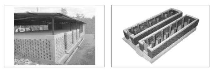
Photograph 6.5 and Figure 6.6: Box composting plant and close-up model of a compost box with plastic door at the front end facilitating emptying (Waste Concern, Bangladesh)
