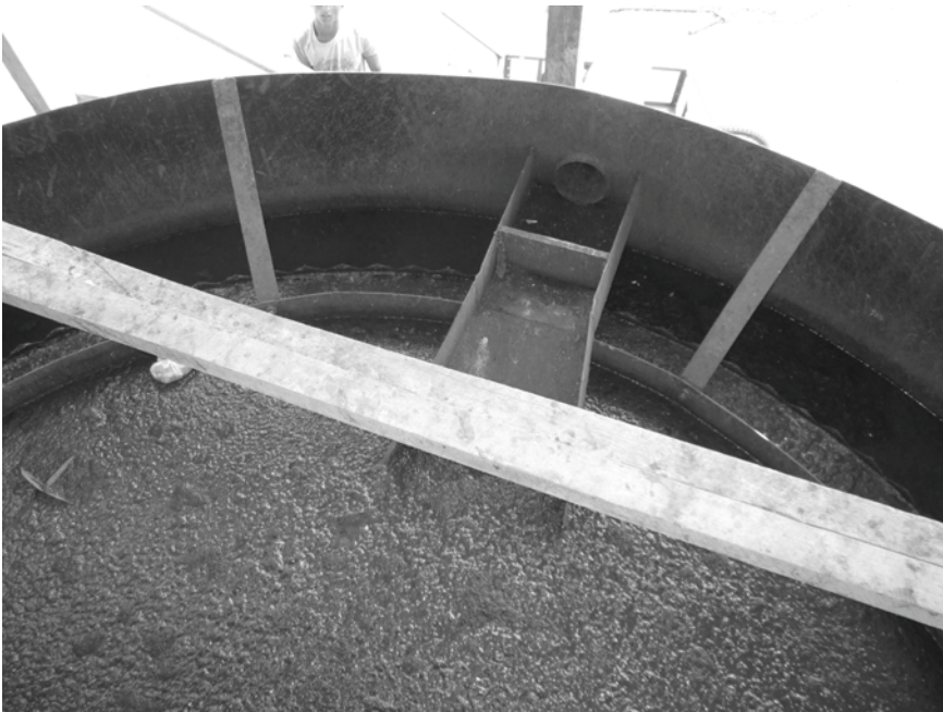
Photo 7.2 Arrangement for scum removal, Sittwe hopper-bottomed tank
