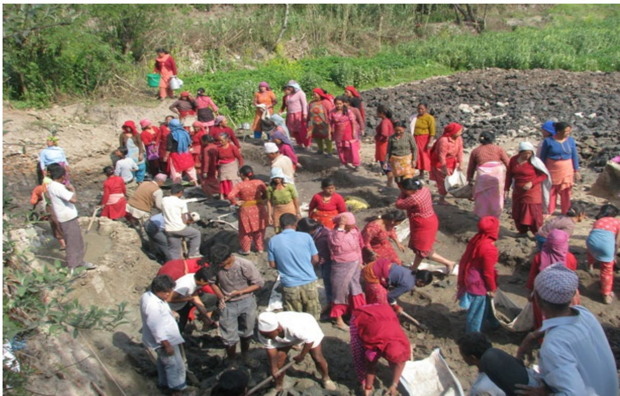
Figure 9: Community self-help efforts - preparing the ground for the decentralised treatment plant (constructed wetland), Nala (Nepal) (Source: M. Sherpa).
