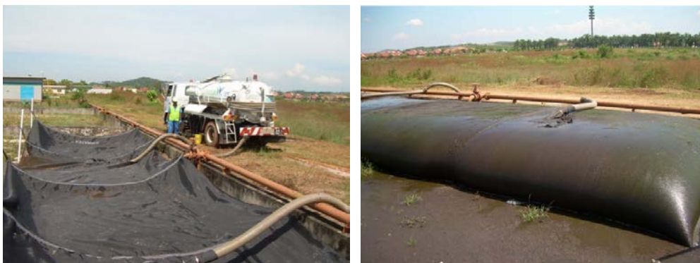
Figure 46: Geo-tube before and after use in Malaysia
