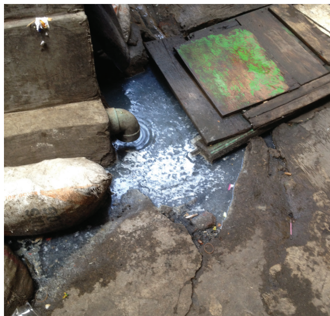
Gray Water Discharge to a Shallow Drainage in Jakarta, Indonesia
