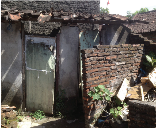
A Public Toilet in Poor Condition in Sangkrah, Solo, Indonesia
