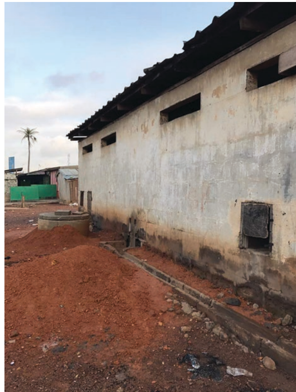
Photo 3.1 • Block Shared by Families That Previously Used Bucket Toilets
