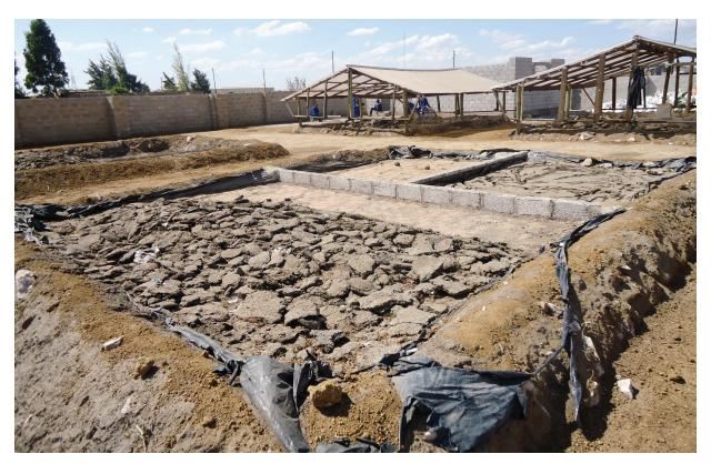
Figure 6: Sludge drying beds
