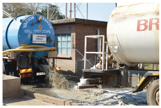
Figure 2: Tankers discharging faecal sludge
