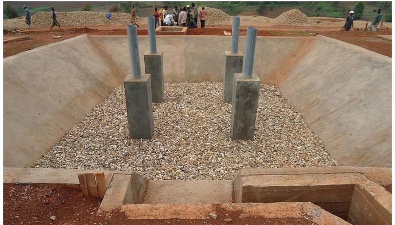
Image: Sludge drying beds under construction. Credit: B. Koelsch
