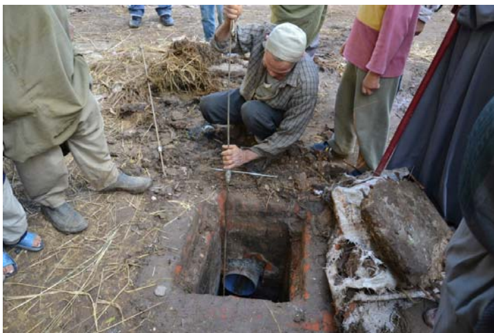
Villager unclogging a sewer pipe (Photo: L. Ulrich)
