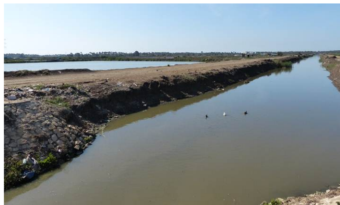
Figure 7: El Malh drain and one of the large aquaculture ponds
