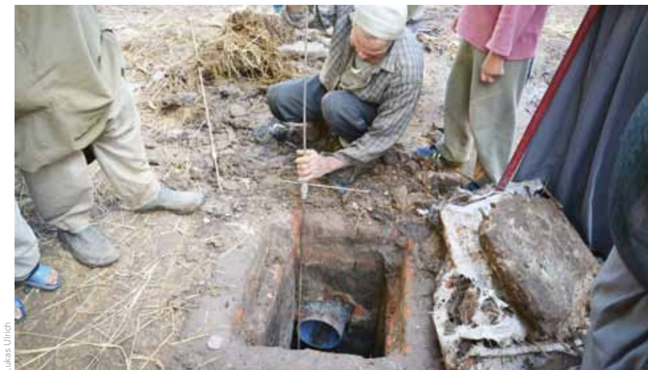
Photo 4: Villager unblocking a sewer pipe.
