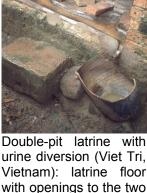
urine diversion (Viet Tri, Vietnam): latrine floor with openings to the two chambers for faeces, a urine diversion channel and a urine pot.
