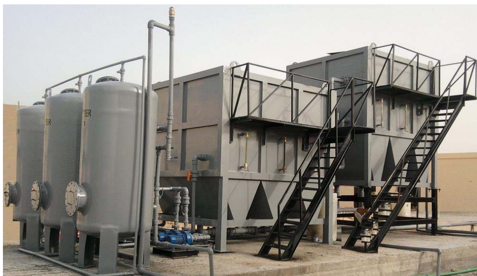
A small-scale prefabricated treatment plant (Al Raed Jetmaster Kimatech 2000)
