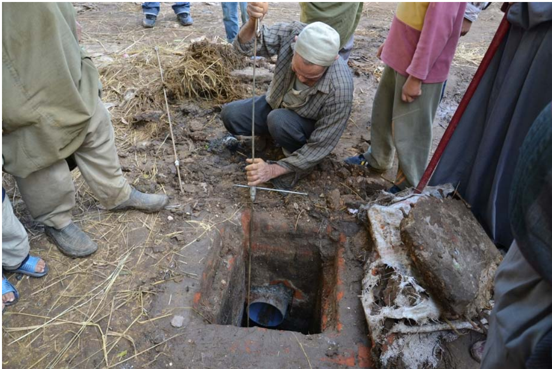
Private stakeholder in charge of unclogging an informal sewer network, Beheira Governorate (photo: Lukas Ulrich)
