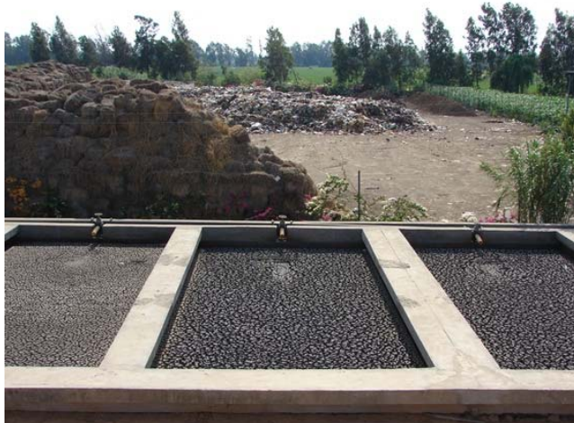
The drying beds and the waste processing site in 2010, including the compost heap (in front), the solid waste to be sorted out (middle) and the sieved compost (back right)
