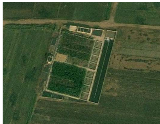
Transformation of the oxidation ponds into constructed wetlands in 2010
