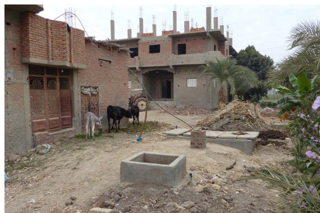
A functioning biogas reactor: the inlet (in front), the biogas pipe (middle) and the bioslurry chamber (back), Fayoum, December 2013
