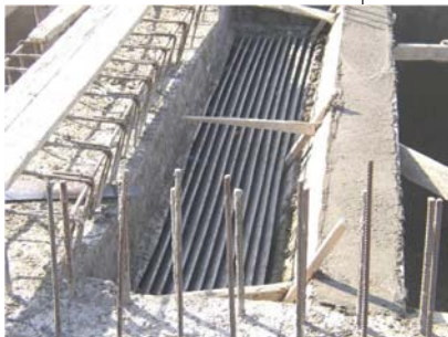
The plate settler during construction (@Tarek Sabry)
