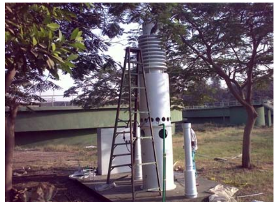
Left: the compact anaerobic tower; below: the pilot in Zenein WWTP, Giza, visited on 18.09.2011
