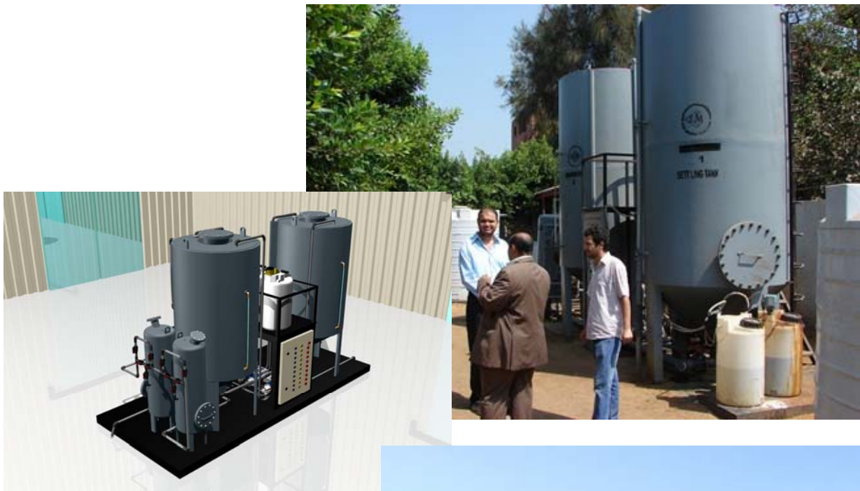
Drawing above: design for about 50 m 3 /day; picture on the right: design for larger capacities - between 300 and 5,000 m 3 /day (courtesy of Al Raed)
